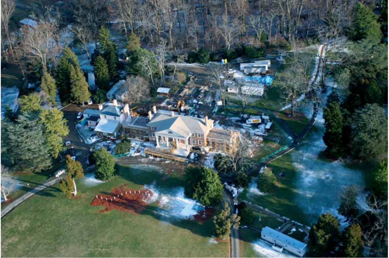
The discovery and restoration of the original Montpelier took five years and $25 million. (Photo by Phil Audibert)
