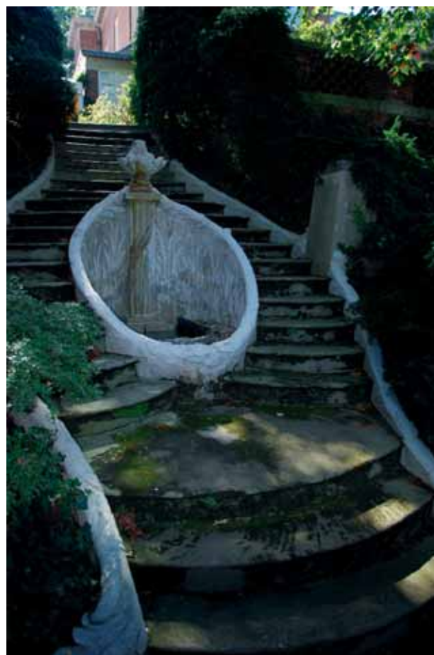
Horseshoe fountain and stair
