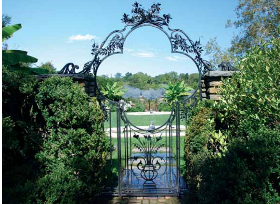
Wrought-iron fountain terrace gate recently reconstructed from the original Farrand pattern
